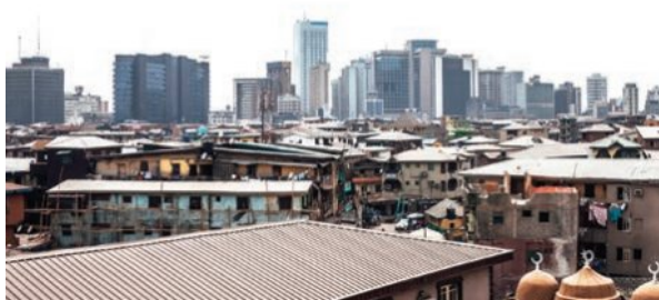
▲ Figure 15.4 Dilapidated buildings sit alongside a modern skyline, Lagos
