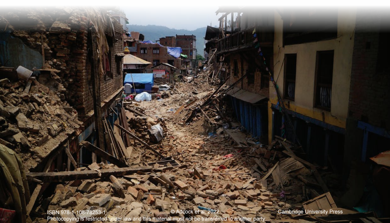
▼ Figure 14.9 Destruction caused by the 2015 earthquake in the Nepalese capital, Kathmandu
