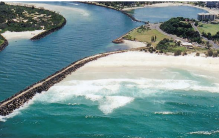
▲ Figure 11.44 Training walls at the mouth of the Tweed River
