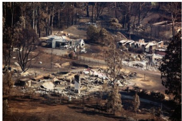
▲ Figure 14.15 Destroyed buildings in Kinglake, one of the many areas devastated by the Black Saturday fires
