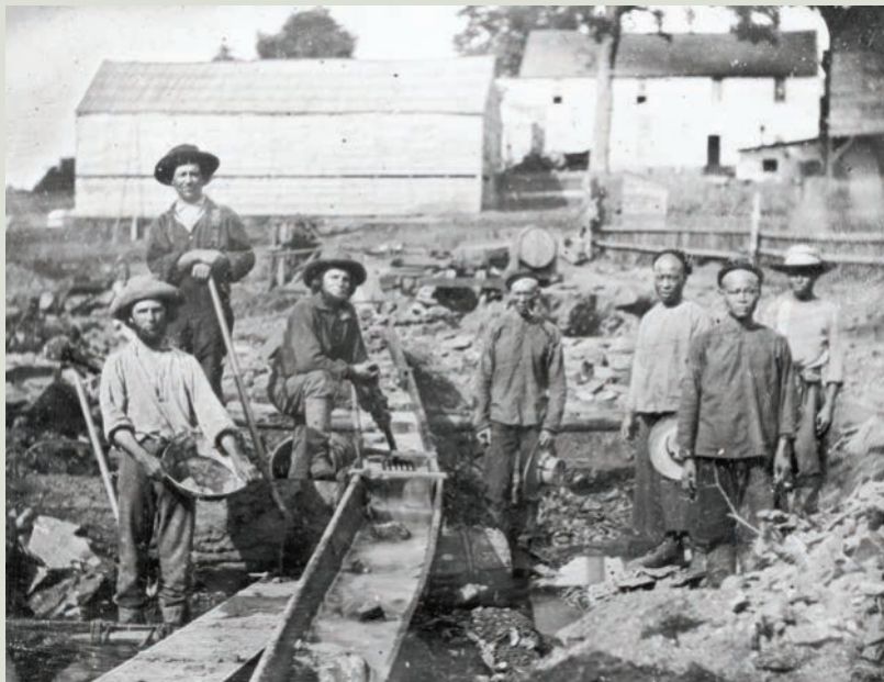
▲ Figure 10.29 Sluicing-box system known as a Californian Pump used by miners in California, 1852
