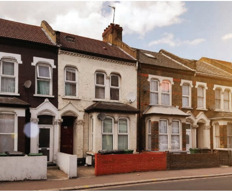
▲ Figure 15.31 High-density terraced houses, such as in Stratford, house London's working class.
