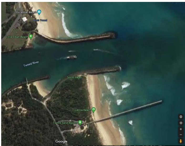
◀ Figure 11.43 Sand bypass system and training walls at mouth of the Tweed River
