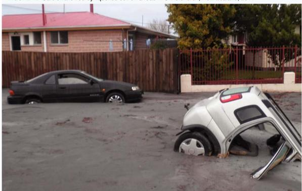
FIGURE 12 Cars swallowed by liquefied soil on a road in Christchurch, New Zealand, 2011
