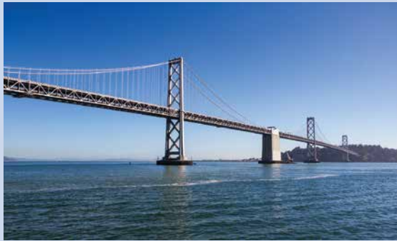
The cables on a suspension bridge form a shape similar to a parabola. Engineers model these curves using equations that include an x^2 term.
