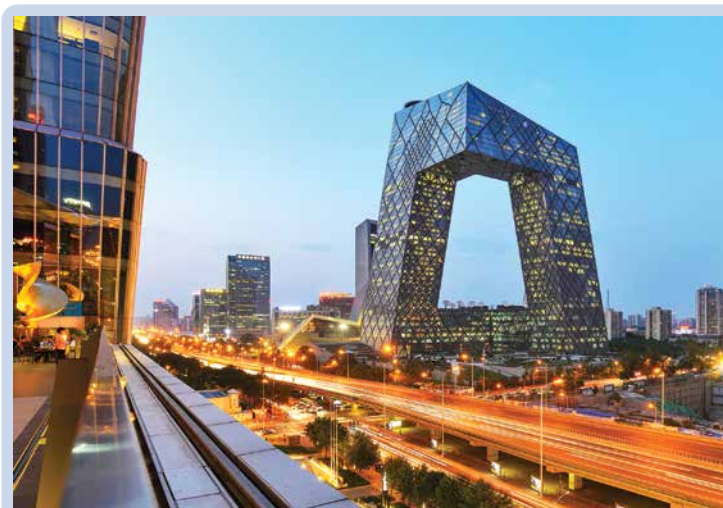
The very 'geometric' CCTV headquarters in Beijing
