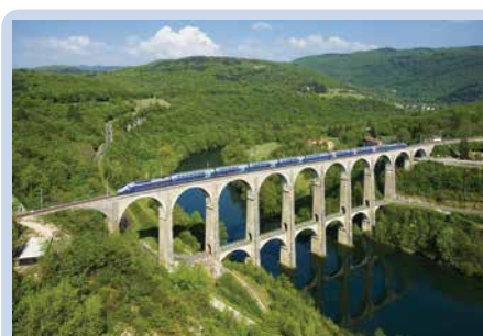
This viaduct in France has a rail and road bridge. Engineers designed its support structure using semicircular arches, radius r , and vertical pylons, height h . Each railway support section has an inside perimeter: P = \pi r + 2h .
