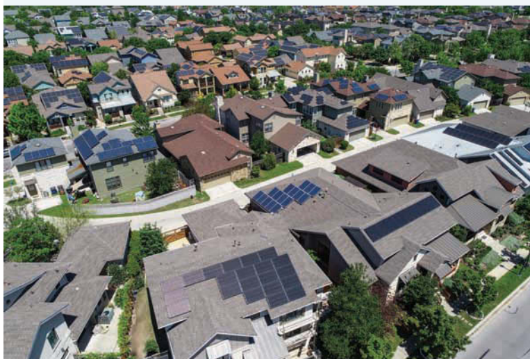
FIGURE 10.20 Solar arrays are often placed on roofs to provide cheap sustainable energy.
