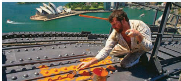
FIGURE 8.23 The Sydney Harbour Bridge is continually painted to protect it from moisture and the air, which would cause its steel girders to rust.
