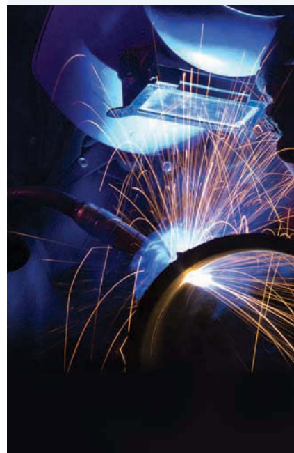
FIGURE 8.27 An oxyacetylene torch is used in construction work.
