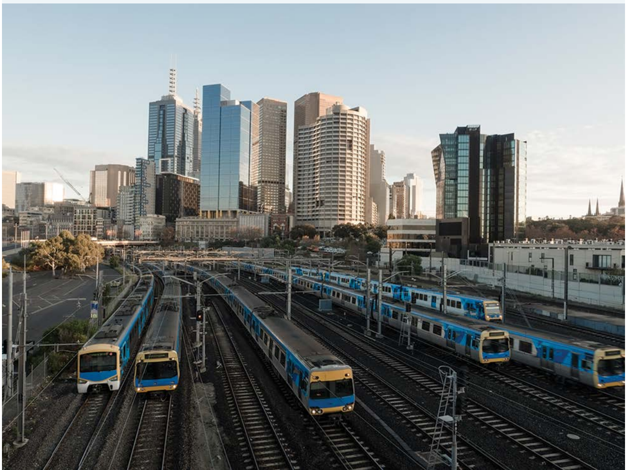
FIGURE 1 Multiple lines facilitate the movement of many trains into and out of central Melbourne.
