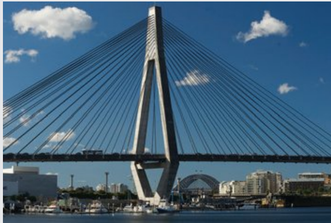
The length of each cable on the Anzac Bridge, Sydney, can be calculated using Pythagoras' theorem.
