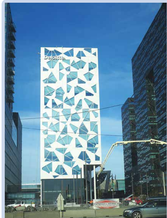
For this high-rise office building in Oslo, Norway, the architect has designed windows with triangular, trapezoidal and composite shapes.
