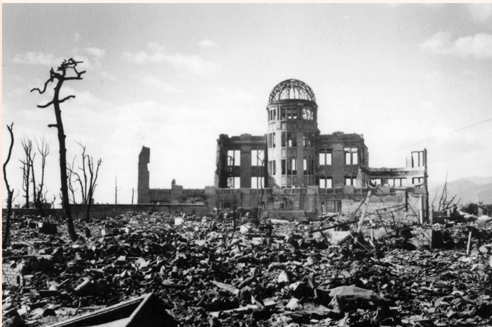
FIGURE 6.23 Atomic bomb destruction, Hiroshima, Japan. Around 90 per cent of the buildings were destroyed, with only a few concrete-reinforced buildings surviving. Some 70 000 people died instantly, with tens of thousands more dying in the aftermath.
