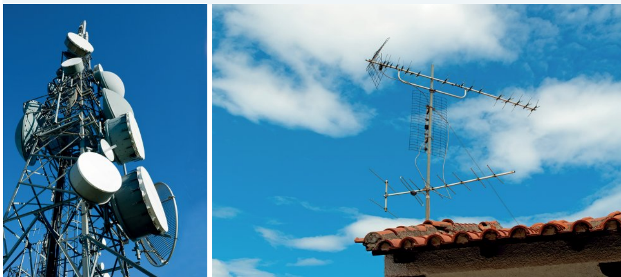
FIGURE 9.65 Compare the sizes of these transmitting (left) and receiving (right) antennae. Why are they different?
