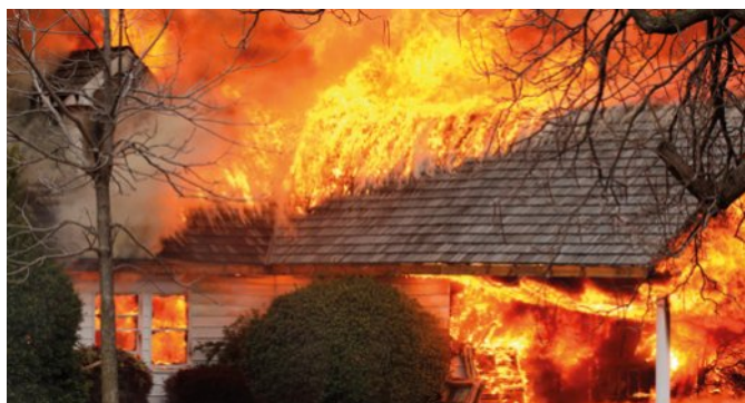
FIGURE 6.3.8 Old or faulty electrical wiring is the most common cause of house fires.
