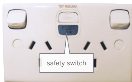
FIGURE 6.3.11 Some power points have their own safety switch.
