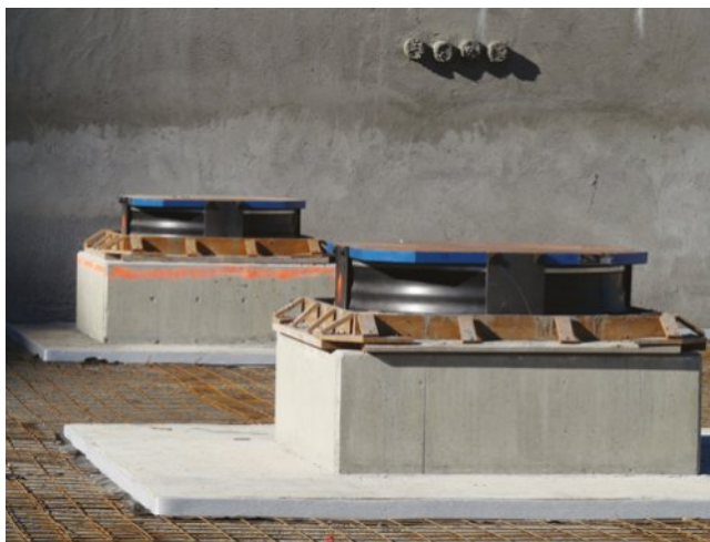
FIGURE 10.3.16 Base isolation involves placing structures such as these rubber bearings under a building.
