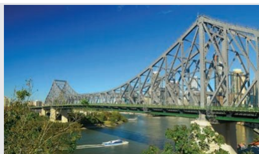
Engineers calculate the angles between the straight structural supports used on bridges such as the angles seen here on the Story Bridge, Brisbane.
