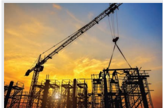
Construction material moved onto a building by a modern crane has undergone a combination of transformations.
