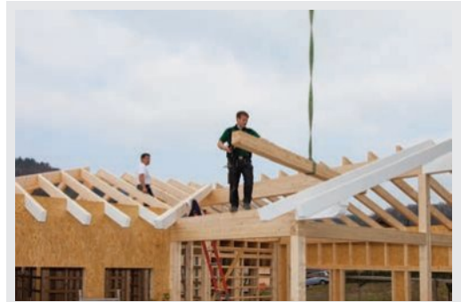
To calculate the number of rafters needed to support a roof, a carpenter first divides the roof length by the required space between each rafter.
