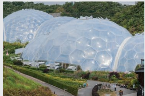
Architects designed these giant domes for plant greenhouses at the Eden Project, England. Steel hexagons, pentagons and triangles support plastic ‘pillows’ full of air that insulate plants from the cold.
