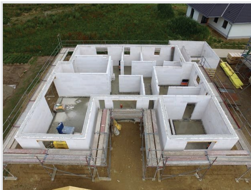
The perimeter of a house is found by adding the lengths of all the outside walls. Scaffolding is required around the perimeter for construction work above ground level.
