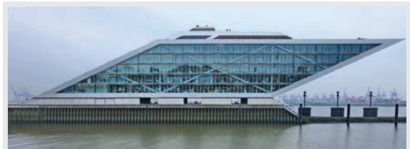
The architect has used a parallelogram to design this office building in Hamburg, Germany. The steel structural supports linking the sides form rhombus shapes and triangles.
