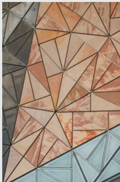
This wall of a building at Federation Square in Melbourne includes many congruent triangles.
