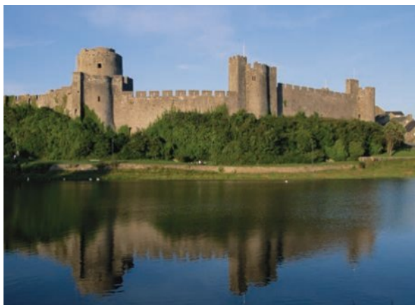
▲ Source 10.52 Bodiam Castle, constructed in England in the fourteenth century
