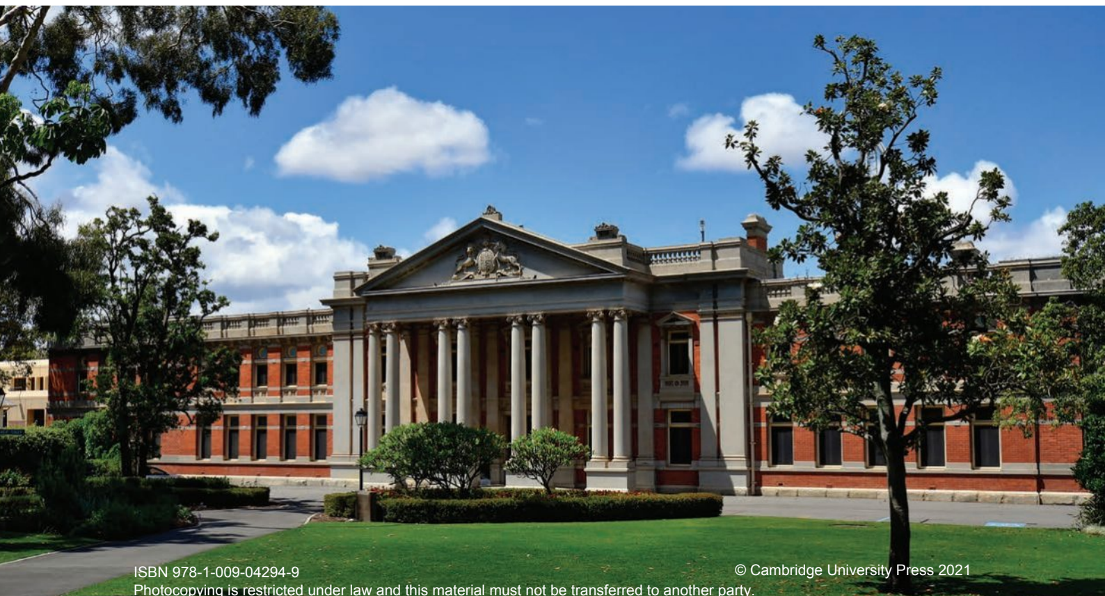
▼ Figure 1.20 The Supreme Court of Western Australia, Perth
