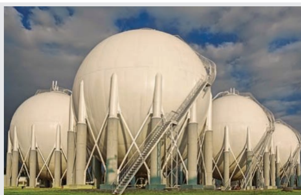
Spherical tanks store compressed or liquid gases for the petroleum and chemical industries. The spherical shape uses the smallest land area for the storage volume and distributes pressure evenly over the sphere's surface area.
