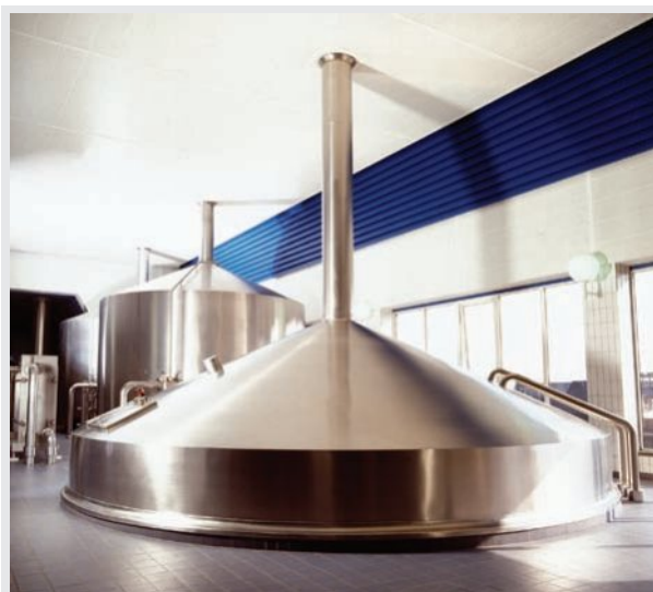
Mechanical engineers and sheet metal workers apply surface area and volume formulas when designing and constructing stainless steel equipment for the food and beverage industries. Cylinder and cone formulas are used when designing brewery vats.
