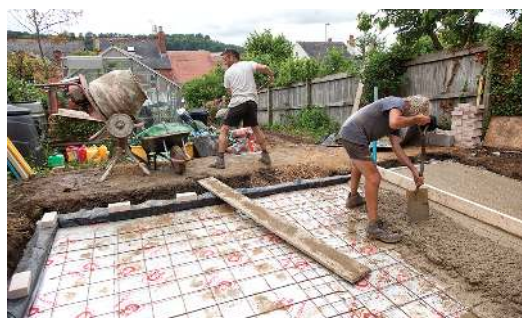
Concrete is made from cement: sand: gravel mixed in a specific ratio.
