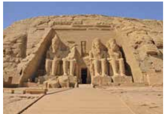
Figure 2.22 Sandstone is a popular building material. This ancient temple of Abu Simbel in Egypt was carved directly into the sandstone rock.
