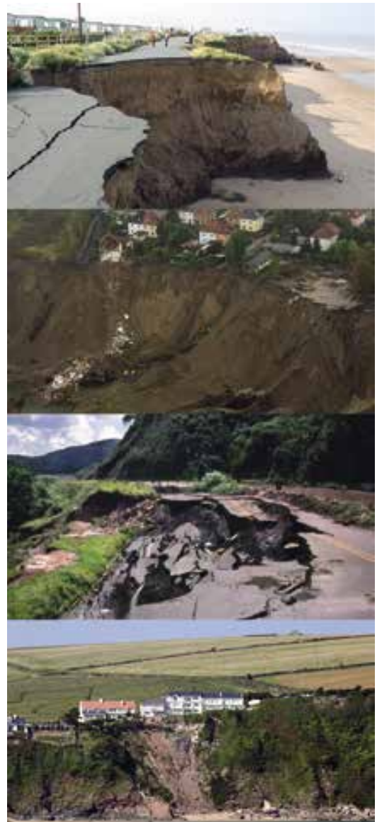
Figure 2.36 Soil erosion can lead to many problems.
