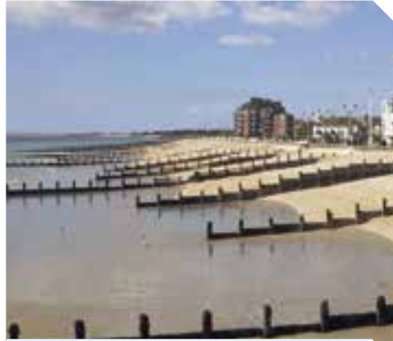
Figure 2.38 Groynes are built on beaches to remove some of the energy of the waves. They protrude from the beach and trap the sand, preventing its erosion.
