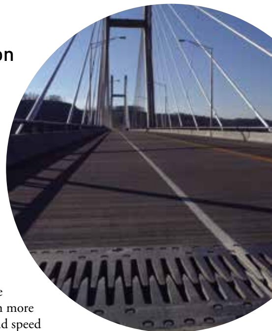
Figure 4.25 An expansion joint in a suspension bridge.
