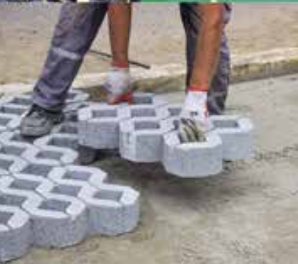
Figure 2.40 New products have been developed that allow water to move through instead of contributing to run-off. This allows the water to be absorbed into the soil and join the groundwater.
