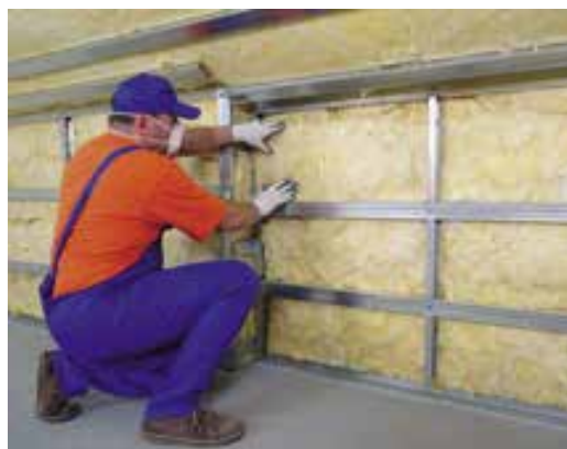
Figure 3.33 Insulation prevents heat energy being transferred between the inside and the outside of the house.
