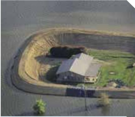
Figure 2.37 Engineers try to minimise erosion by controlling the flow of water with dams and levees.
